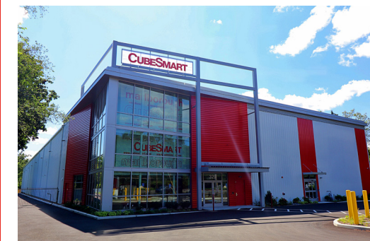
BETCO multistory installation: Marlborough, MA
