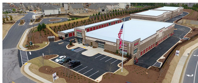
BETCO multistory installation: Johns Creek, GA
